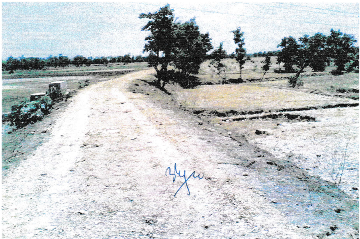
Murum Topping and Repair of Bund Line.
