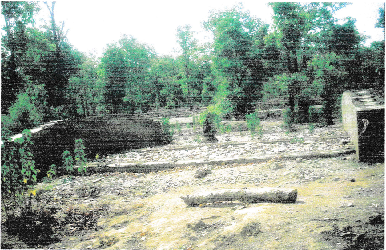
New construction of Flush Bar Type Waste Weir.
